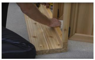
Place the bottom Shelf on a flat surface with the predrilled holes on the bottom.
