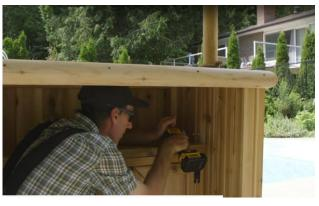
Secure the assembled bar to the T posts from the inside using a 2 ½" (64mm) screw.
