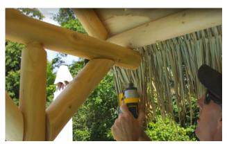
Once the roof is even on each end, pre-drill holes in each of the T posts lining the hole up with the roof bottom side plates.
