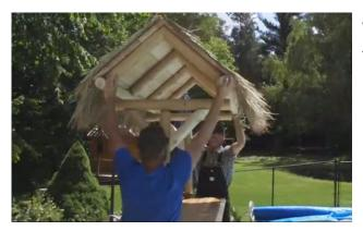
With at least 2 people, lift the assembled roof onto the top of the bar posts.
