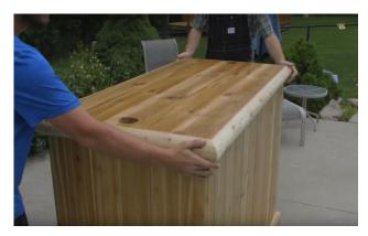
With a helper, place the bar top on top of the assembled frame.
