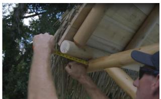
Using a tape measure, ensure the overhang on each end of the roof sits even.
