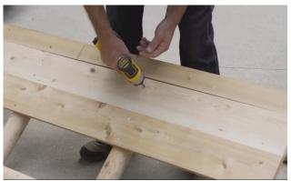
Install the roof boards (tongue & groove) working your way down each side of the roof.
