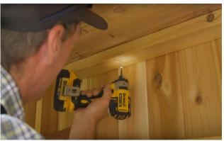
Secure the long front wall to the bar top from underneath with 2 ½" (64mm) screws.
