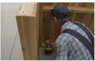
Holding the walls flush together, secure them together using the provided 2 ½" (64mm) screws from the inside of the long front wall into the short side walls.
