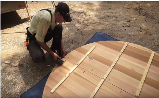
Line up the 2 halfmoon floor pieces so the edges are flush, Screw the 2 halves together using 2 1/2" (64mm) screws on both sides of the floor seam.
