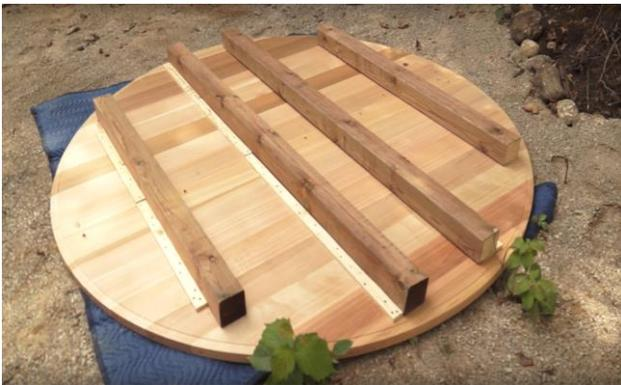
Place the Long Floor Supports against the inside guides and the short Floor Supports against the outside guides.
