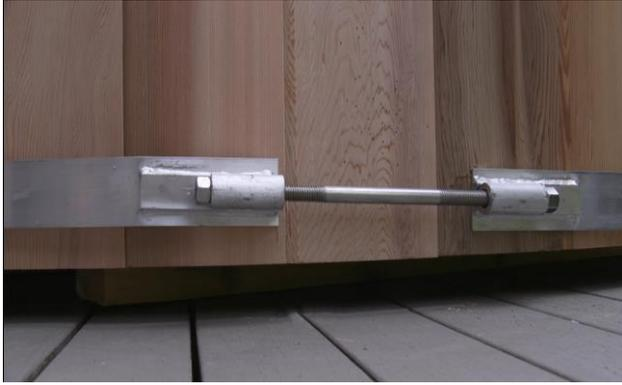
Wrap the second band around the bottom of the shower and attach in the same manner as the top band.
