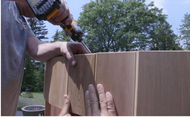
Make sure the assembly is flush at the top and screw into the door side staves.
