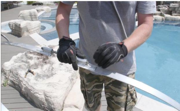
Bring the 2 ends of the first band together and connect them with the threaded bolt and a nut on either end.
