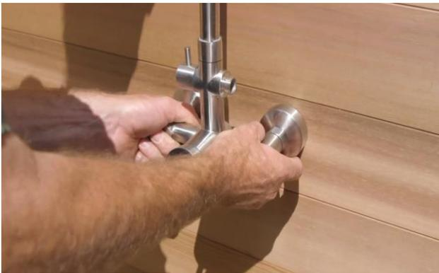
Place the adapters through the drilled holes.
