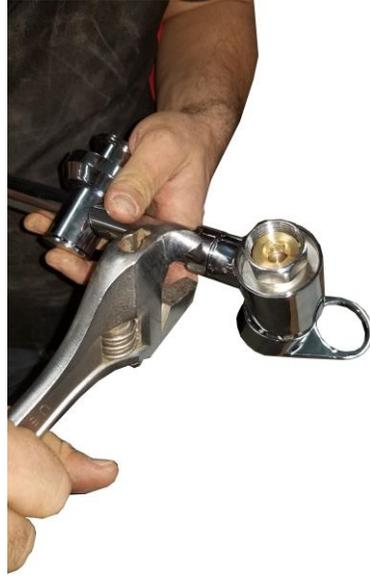
Thread the handle assembly (C) onto the shower pole (B).
