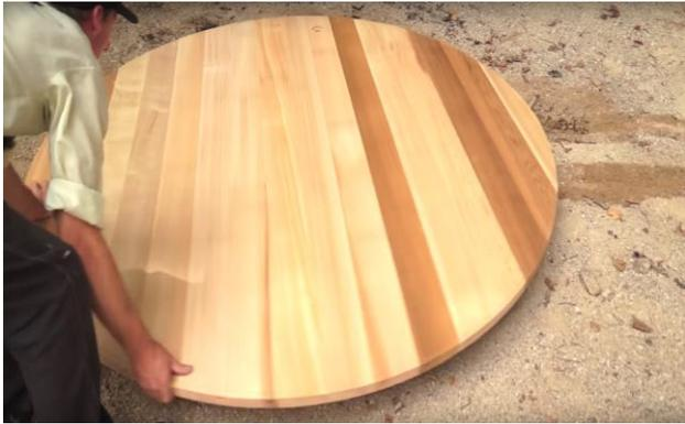
Once the floor supports are secure to the underside of the floor, flip the floor over and position it in its proper place on the foundation.
