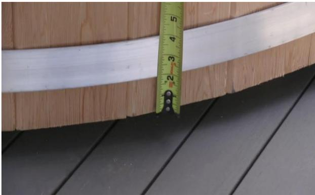
The bottom band should be 2" (51mm) from the edge of the stave to the bottom of the band.
