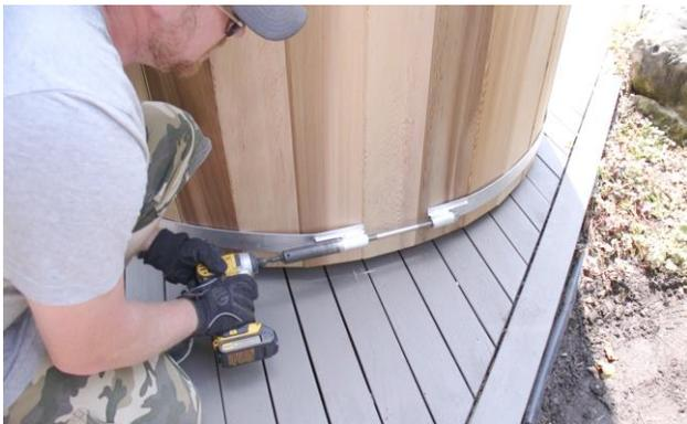
Using a wrench or impact driver, tighten each band a little at a time starting with the bottom band.
