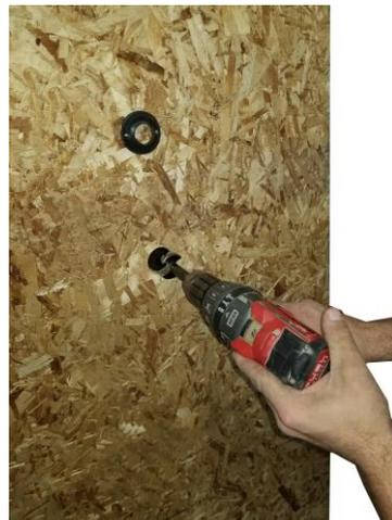
Measure the distance from the bottom support flange to the hose hook up on the handle and drill a hole in the shower large enough for your plumbing to go through to attach to the handle assembly.
