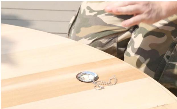
Insert drain into the hole in the floor and tighten firmly.
