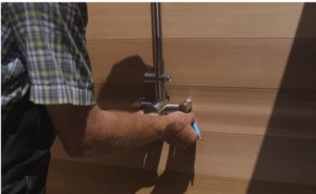
Center the bottom of the fixture and mark where to drill your holes for the water connections.
