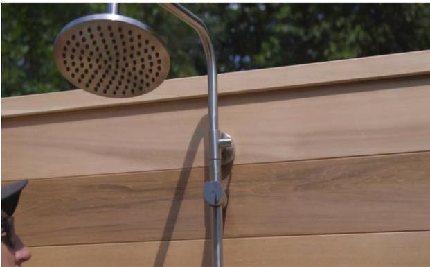
Place the mounting cover over the bracket and attach the assembled premium shower fixture.
