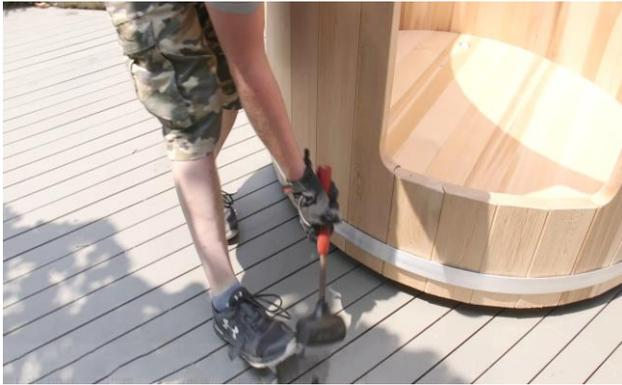
To make installation easier, have a helper walk around the shower hitting each stave with a firm rap on the bottom strap while you are tightening the band.
