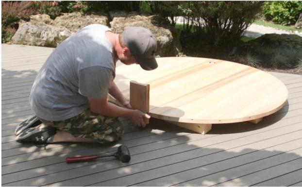
Attach the short bottom staves on the opposite side of where the drain is located.
