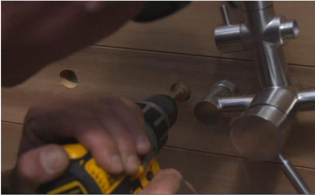
With your hole locations marked, slide the fixture to the side and drill through the board using a bit large enough that the adapter will fit through.
