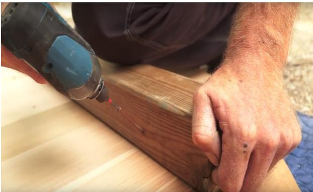
Using 2 1/2" (64mm) screws, secure the floor supports to the floor sections as shown.
