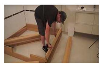
Once the front and back staves are installed, insert another side wall stave on either side.
