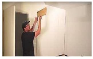
Insert a front wall stave as shown. These will be the shorter staves to go on either side of the door.
