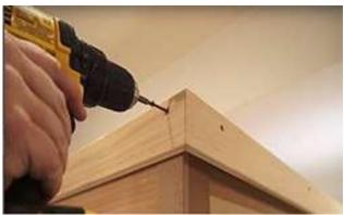
Line the front roof trim with the side trim ensuring they are flush and secure with 1 ½" (38mm) screws.
