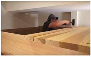
Install a roof stave into the roof trim on the top of the sauna by sliding the grooves of the stave over the front and back walls and tapping the roof stave flush into the roof trim.
