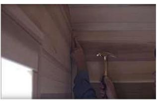
Measure each of the 4 corners inside the sauna and cut the interior trim pieces accordingly.
