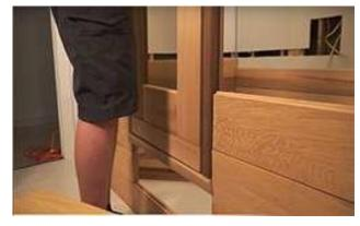
Carefully slide the groove of the door frame into the front wall staves.
