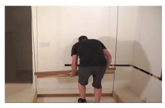
Place a side wall stave on either side using the same method as in the previous steps.
