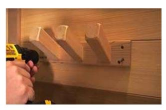
Install the towel hanger at the desired height on the outside of the sauna and secure with 1 ½" (38mm) screws.
