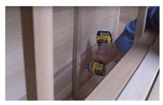
Secure the middle brackets to the back wall using 2  $\frac{1}{2}$ " (64mm) screws in the pre-drilled holes.
