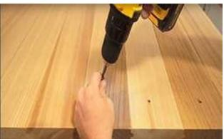
Secure the roof staves into the front and back walls using 2 ½" (64mm) screws.
