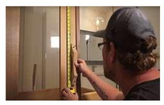
To make it easier to get in and out of the sauna during assembly, when you have the walls built around halfway to the top of the sauna, center the outer door handle (small) at the desired height on the outside of the door and secure with 2" (51mm) screws in the predrilled holes.
