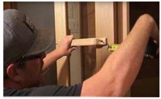
Install the inner door handle (large) centered horizontally on the inside of the door at the desired height and secure with 2" (51mm) screws.
