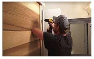
Secure the outer trim pieces to the outside corners of the sauna using  $1 \frac{1}{2}$ " (38mm) screws.
