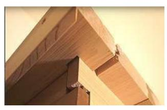
When you reach the opposite side of the roof, tap the remaining roof trim piece flush into position using the rubber mallet.
