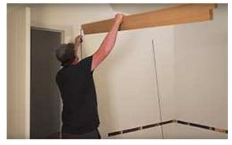
Slide the front and back bottom staves over the threaded rod and slide down.
