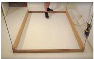
Once the 2 sides and the front and back staves are slid down over the threaded rods, square up the base.
