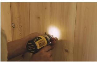
Install the two  $\frac{1}{2}$ " x 1  $\frac{1}{2}$ " (6mm x 38mm) hex head lag screws (supplied with the heater) into the holes.
