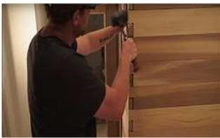
If necessary, use the rubber mallet to correct any warping or slightly out of place staves.
