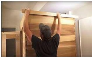
Place the roof trim on top of the side wall.
