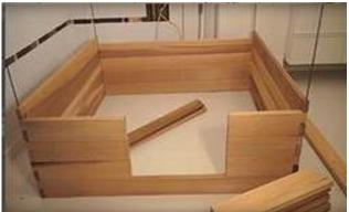
When you complete the 4<sup>th</sup> row on the front wall, it is time to install the door.
