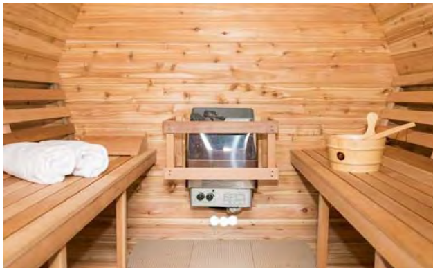
Inlet under electric heater on Back wall
