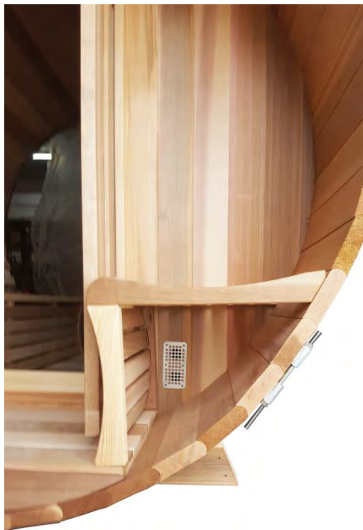
Inlet Vent on front wall
