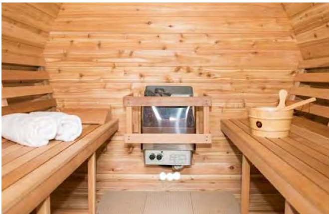
Inlet under electric heater on Back wall
