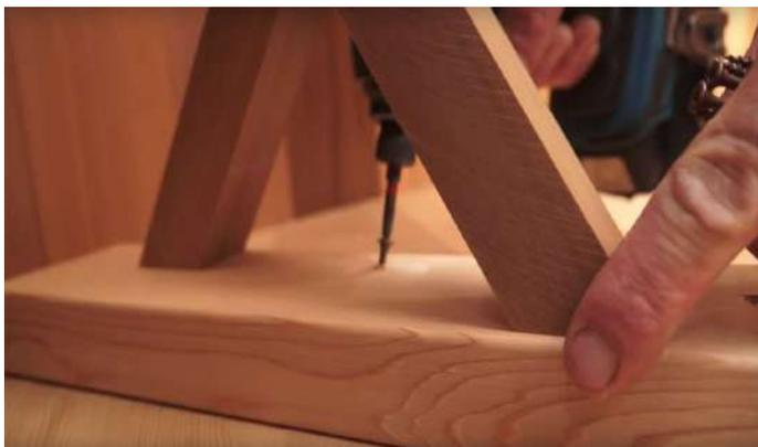
Fasten the bench supports to the tub floor using 2 1/2" screws.
