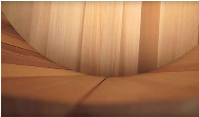
You must avoid having the floor seam line up directly with any of the seams between the staves.
