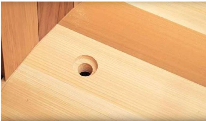
You can install the floor drain at this time in the recessed hole in the floor.
