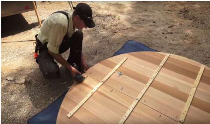
Line up the 2 pieces so the edges are flush, insert a 2 1/2" Kreg screw into the edges on both sides of the floor seam.
