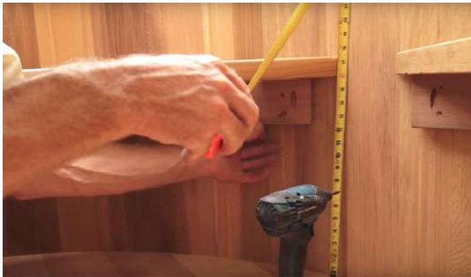
Measuring 17 1/2" from the floor to the top of the bench on each end should make sure that the bench is level.
