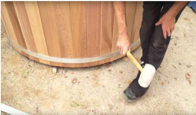
Work your way around the tub, hitting each stave with a firm tap on the bottom band.
