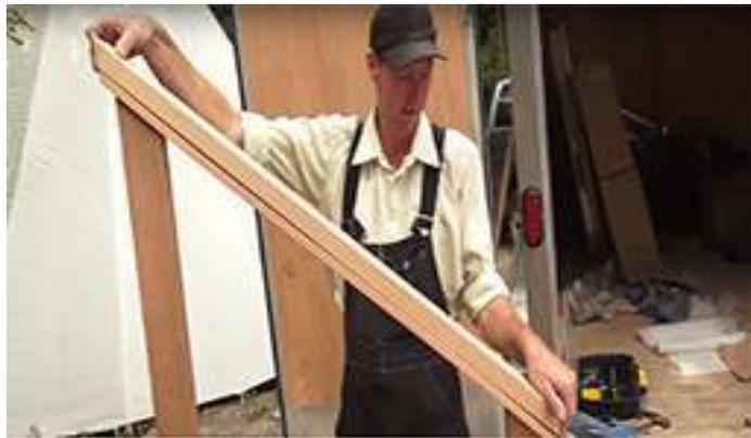
Make sure the bottom edge of the top railing is flush on the ends to the bottom railing and secure up through the bottom railing using 2" screws.
