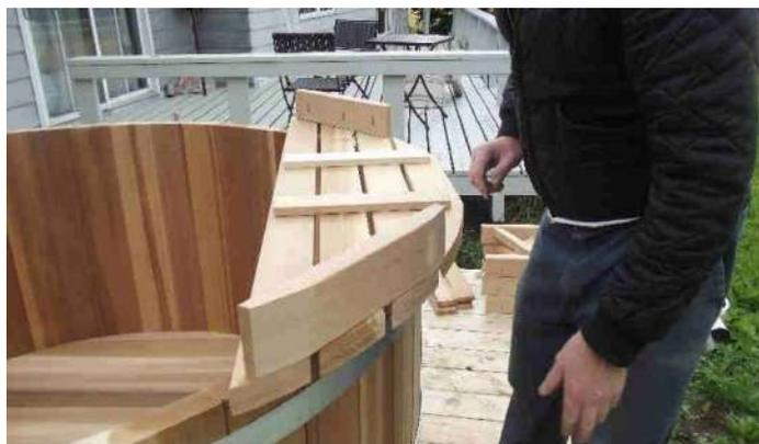
Make sure that the bench brackets are flush with the ends, and about  $\frac{3}{4}$ " back from the front edge of the benches.
