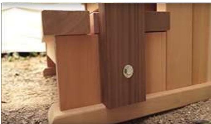
Attach the railing supports on the 3<sup>rd</sup> and bottom steps where the step is recessed and secure with the provided nut and bolt through the pre drilled hole.
