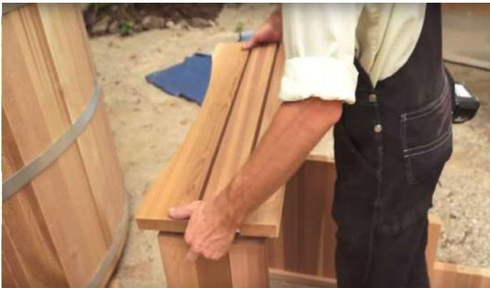
Lay the top step on the top of the stairs with the curved side facing the hot tub.
