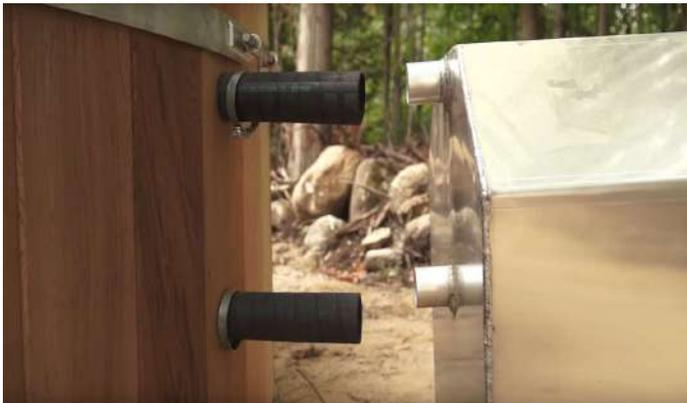
Slide the heater hoses onto the outer side of the heater hose fittings and secure with gear clamps.
