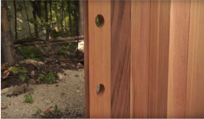
Insert the stave with the holes in it in line with where the heater will be.
