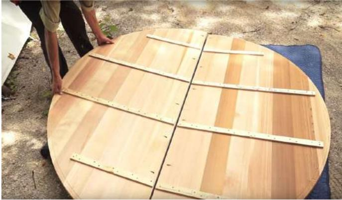
To protect the wood during installation, lay the 2 floor pieces upside-down on something soft like a blanket.
