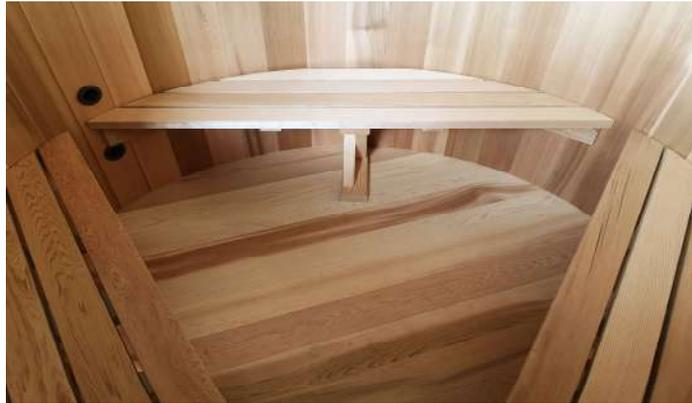
The Cedar Hot Tub has 3 benches. They each sit on two end brackets attached to the walls, and one support in the middle attached to the floor.
