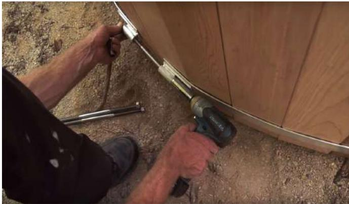
Tighten the nuts with a 3/4" wrench until the band is just snug enough so that it will stay in place.
