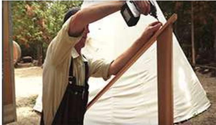
Center the bottom piece of the railing on to the railing supports and secure with 2" screws.
