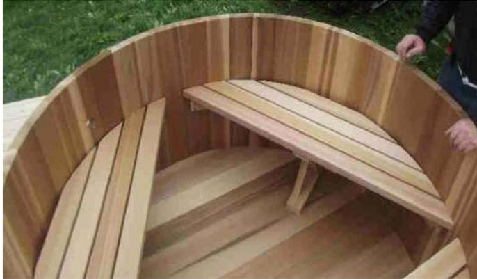
By trial and error, position the three assembled benches into the hot tub spacing them equally apart.
