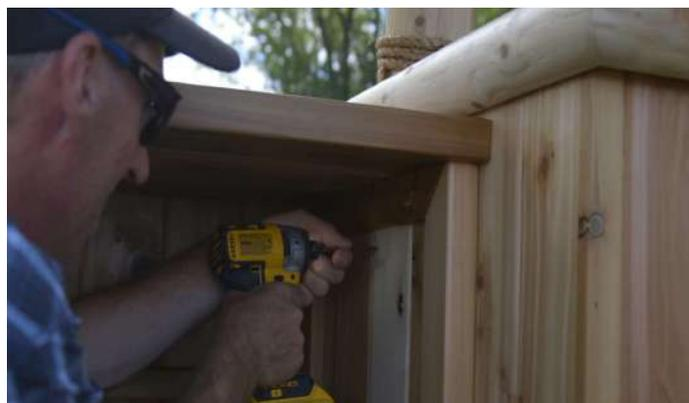
Secure the bar posts from the inside of the base using the provided 3" (76mm) wood screws.
