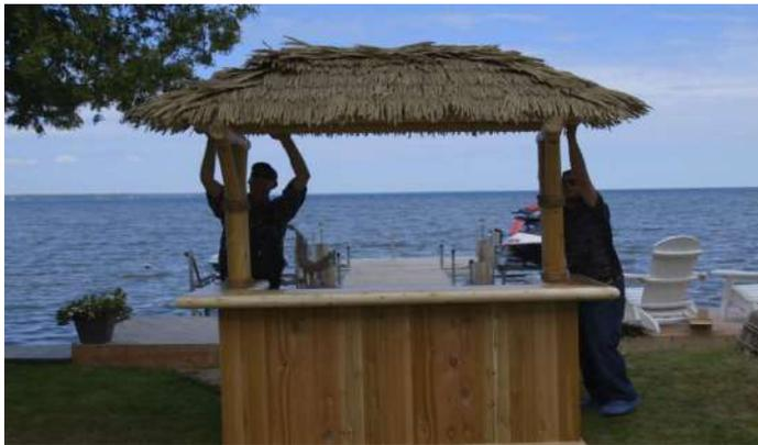
With a helper, place the roof up onto the bar posts.
