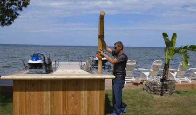
Insert the bar posts into the holes on the top of the tiki bar.
