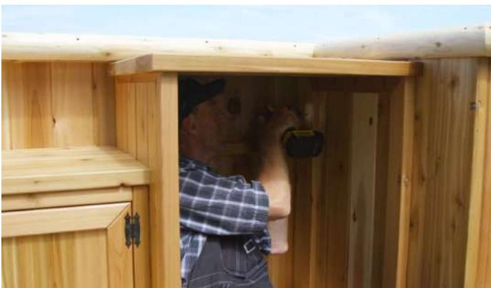
Repeat the process by fastening inside the mini fridge compartment to the tiki bar base using 2 ½" (64mm) screws.
