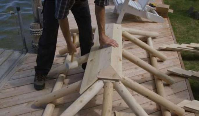
Starting on one of the sides, insert the shortest board up tight to the roof cap.
