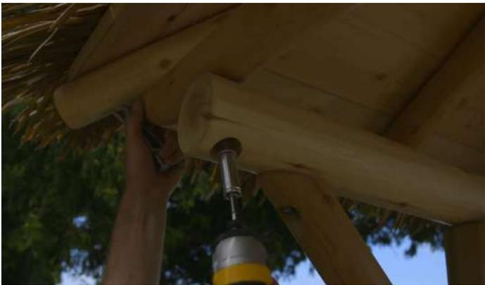
Secure the bar posts to the assembled roof using the supplied lag screws.
