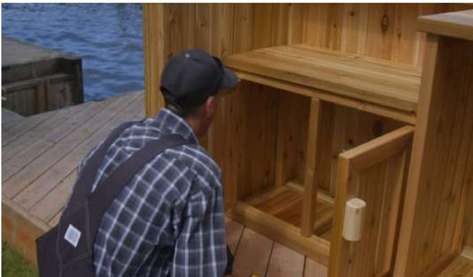
Secure the frame on the inside of the bar cabinet to the tiki bar base using 2 ½" (64mm) screws.
