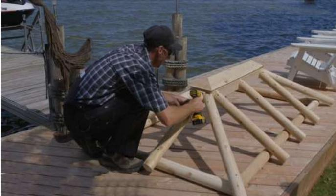
Center 1 roof support on the end and secure as in the previous step.
