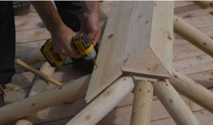
Secure the roof boards into the roof supports with the provided 2" (51mm) screws.
