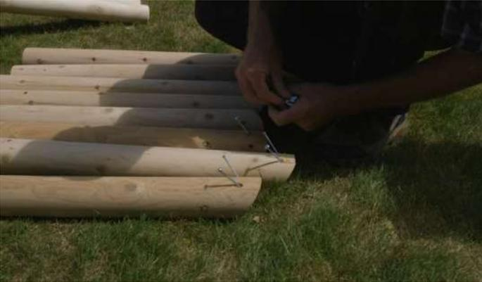
To make installation easier, pre place 3" (76mm) screws into the ends of the roof supports.
