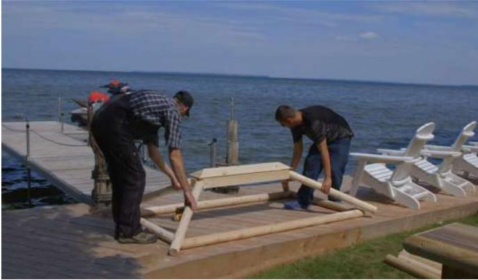
Center the roof cap assembly on top of the roof frame.
