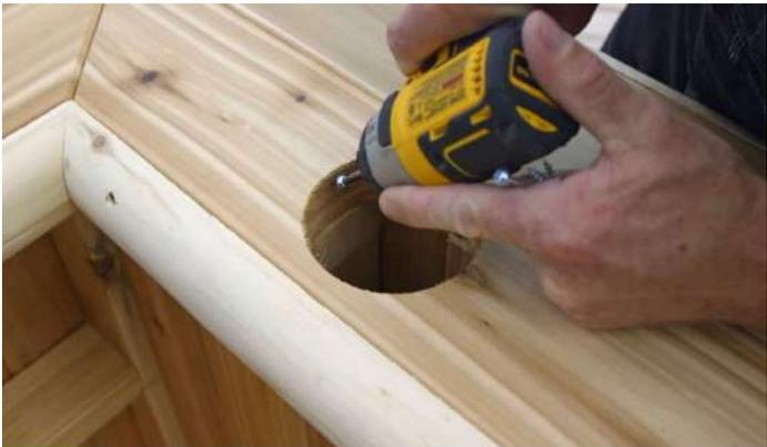
If the roof option is chosen, secure the bar top to the base through the post holes.
