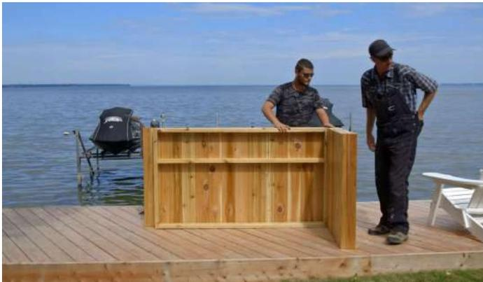
Slide one of the side wall pieces flush into the front wall.
