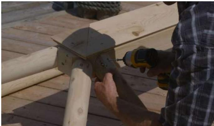
Position one of the shorter supports flush to the side and top of the side of the roof cap and secure with 3" (76mm) screws.
