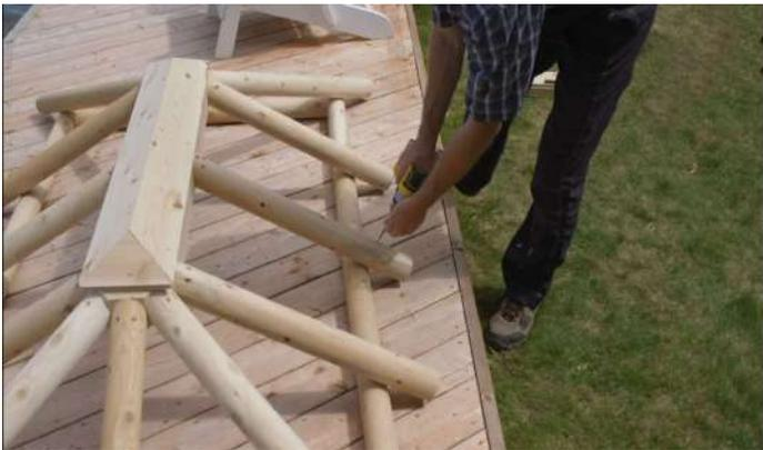
Screw the bottoms of the roof supports to the roof frame using 3" (76mm) screws.
