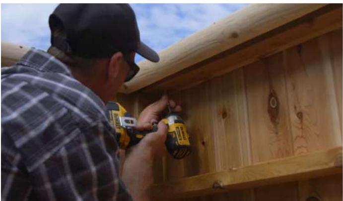
Secure the base to the bar top using the provided 2 ½" (64mm) screws from the inside of the front wall up into the bar top.
