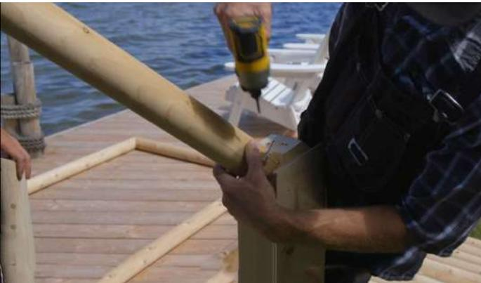
With assistance from a helper, hold the corner roof support flush to the corner of the roof cap assembly. Secure the post to the assembly with 3" (76mm) screws. (2 screws per corner)
