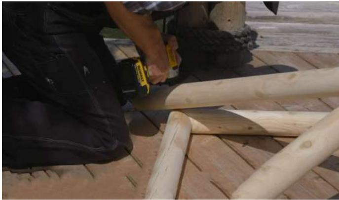
Screw the corners of the roof supports to the roof frame using 3" (76mm) screws.
