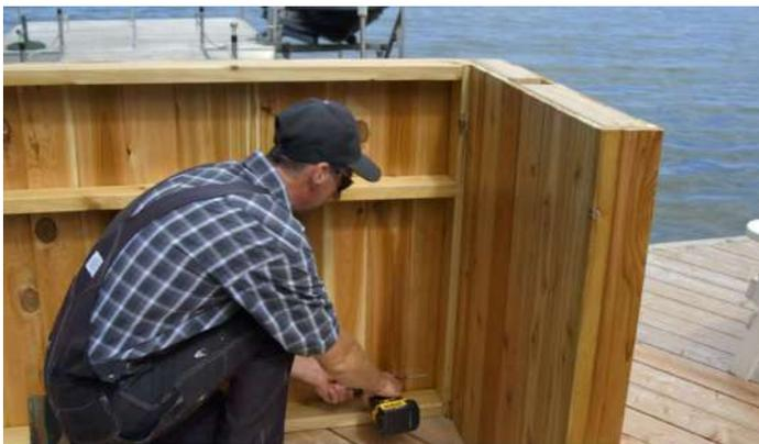
Holding the walls flush together, secure them using the provided 2 ½" (64mm) screws from the inside of the front wall into the side wall.
