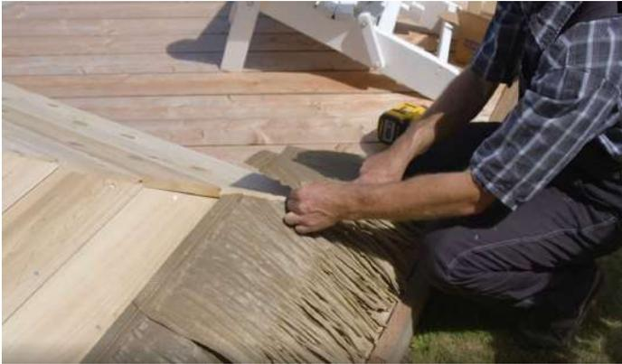
When you get to the end of the roof, cut off the excess thatch with a utility knife.
