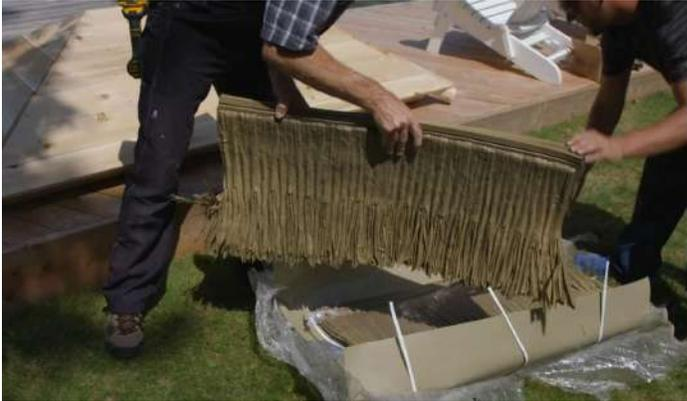
Place the thatch onto the roof with the synthetic palm leaves hanging over the bottom as in picture.
