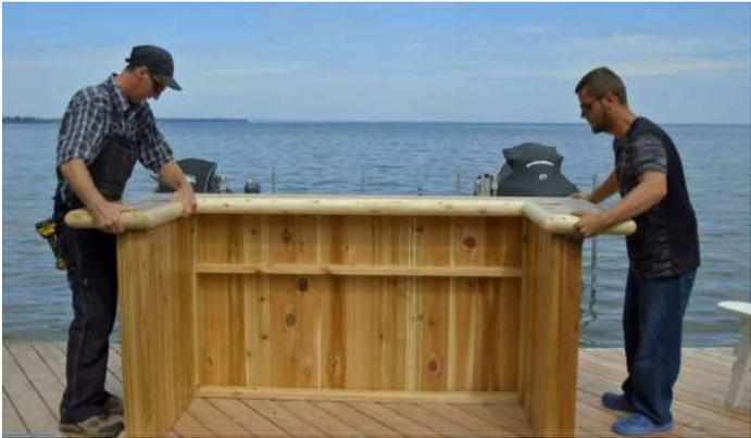
Place the bar top onto the assembled bottom base.
