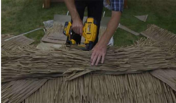
Overlap the 2 cut pieces back to back then secure into place with staples.
