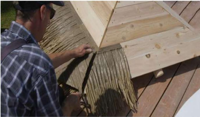
Use the cut off piece to start the first row on the short side. Cut the excess off the corner in the same manner.
