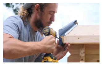
Fold over the ends of the metal trim pieces and secure with the included black short screws.
