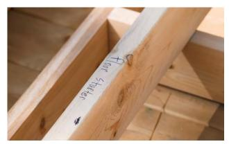
To start the assembly of the floor, locate the stave that is labelled "Floor Starter"
