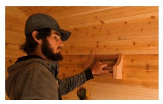
Install the optional shelf at the desired location and secure with 2 - 1 1/2" (38mm) screws.
