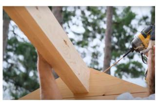
Secure each end with a 5" (127mm) screw on each side of each triangle piece.
