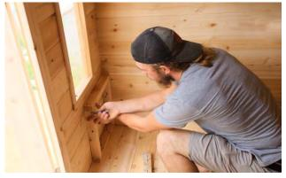
Place the small bench support against the wall and mark the top and the front as in previous steps.
