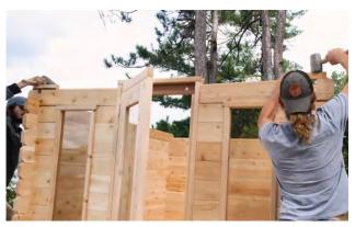
Place a medium length front wall stave above each window and secure using a 5" (127mm) screw into each notch.
