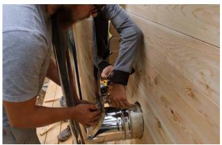
Attached assemble chimney pieces to the "T" coming out the back of the sauna and secure with a support band.
