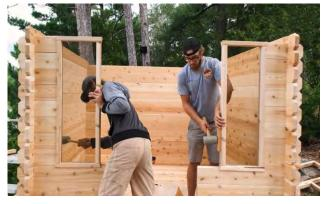
Place your windows onto the front wall and ensure the staves are fully inserted into the grooves.
