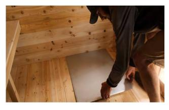
Place the heat shield on the floor where the stove will be.
