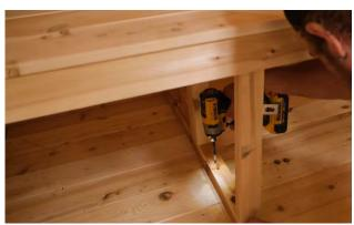
Screw the bench supports to the floor and back wall using 2 ½" (64mm) screws.
