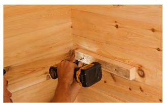
Mount one of the wall mount bench brackets flush to the line on the upper bench and secure with  $3 - 2 \frac{1}{2}$ " (64mm) screws.
