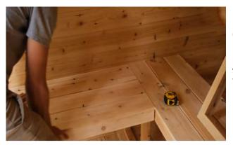
Place the bench on the supports and secure with 2  $\frac{1}{2}$ " (64mm) screws.
