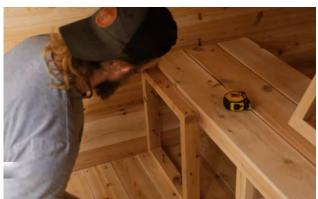
Screw the bench support to the benches and side wall using 2 ½" (64mm) screws.
