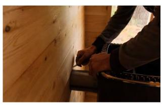
Place the short metal pipe into the back of the stove and mark it where it meets the wall.
