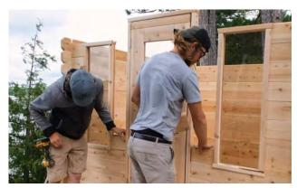
Slide all the small front wall staves between the door and windows and ensure they are tight to each other by tapping with a mallet.
