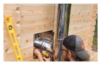
Overlap the top half of the exterior chimney shield and secure with provided screws.
