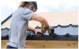
Overlap the panels one ridge and continue securing to the roof to the other side of the sauna.
