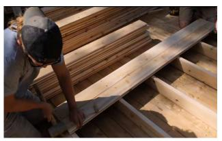
Align the next floor stave up to the edge of the first one and tap the tongue into the groove.
