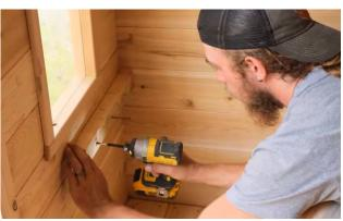
Mount the remaining wall mount bench bracket flush to the line of the bench and secure with 3 - 2 1/2" (64mm) screws.
