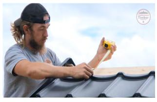
The last row of roof shingles will be precut to size.
