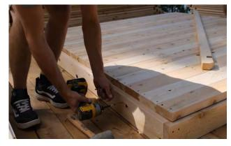
Place 3 -3" (76mm) screws into each of the side supports.
