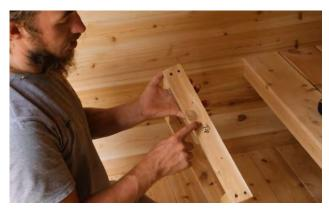
Place the small bench support on the other end, make sure the side labelled "top" is upward.
