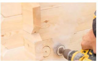
Mark the vent inlet hole positions on the side wall of the sauna, next to the stove, and drill out with a 2" (51mm) hole saw.
