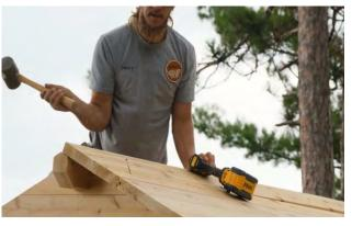
When you reach the top of one side, use the wide stave without the groove on the top.
