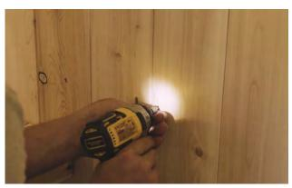
Install the two 1/4" x 1 1/2" (6mm x 38mm) hex head lag screws (supplied with the heater) into the holes.
