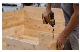
Place a short front wall stave on either side of the front wall and .secure with a 5" (127mm) screw in each of the notches.
