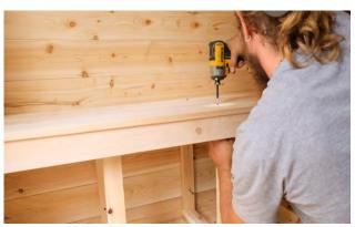
Line up the supports and secure the bench to the supports and the supports to the floor and side wall in the same manner as previous steps using 2  $\frac{1}{2}$ " (64mm) screws.
