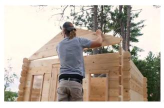
Place the front and rear triangle front pieces onto the sauna.
