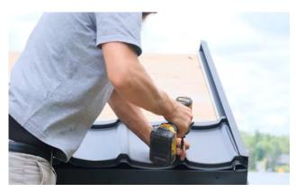
Start applying the metal shingles by sliding the shingle under the side metal trim piece and flush with the edge of the side trim and then secure using the included roofing screws.
