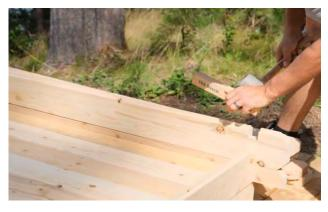
Now place a full-length stave at the rear of the sauna and tap the tongue and groove together to make sure it is tight and secure with a 5" (127mm) screw into the notch at either end.
