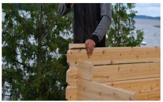
Repeat the process of placing and securing the sides, back wall staves and short front wall staves until the short staves are 8 staves high.
