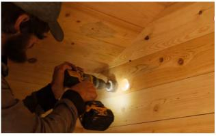
Mark the vent outlet hole position high up on the back wall.
