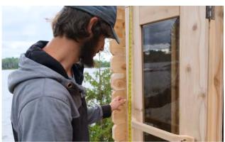
Install the inner door handle (large) horizontally at the desired height. Ensure the handle is level and secure using 2 – 2 ½" (64mm) screws in the pre-drilled holes.
