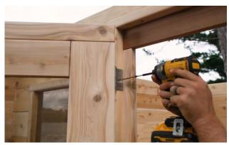
Place a 3" (64mm) screw through the middle hole on the 2 hinges and then centered in the frame between the 2 hinges.
