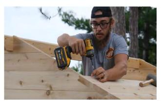
Start placing the roof staves going up the roof and tap into each other, secure with 2 - 3" (64mm) screws into each end.
