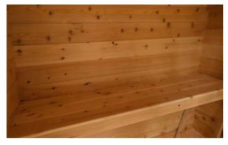
Place the top bench onto the supports and secure with 2 ½" (64mm) screws into the wall mount bench brackets.
