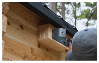
Mark the center of the 3<sup>rd</sup> support piece and install the chimney support bracket centered on this mark with the included lag screws.
