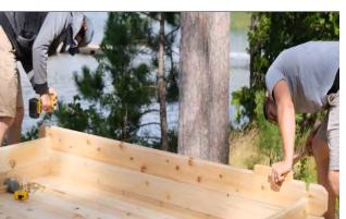
Continue this process using a full-length stave at the rear of the sauna and tap the tongue and groove together to make sure it is tight and secure with a 5" (127mm) screw into the notch at either end.
