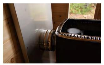
Place the chimney through the hole, then through the heat shield (hole towards the bottom), then into the stove.
