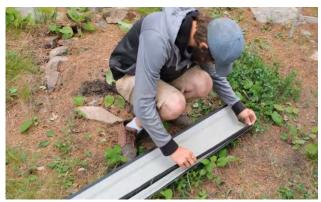
Reveal the adhesive side of the M-seal and apply it to the inside edges of the roof ridge cap.
