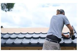
Continue adding the shingles up the roof overlapping the previous row securing with roofing screws on every ridge until you get to the last row needed.
