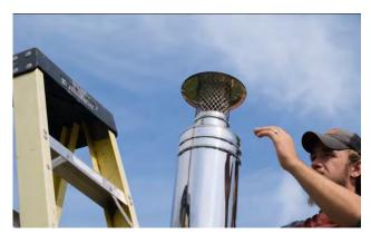
Install the cap on the top of the assembled chimney.
