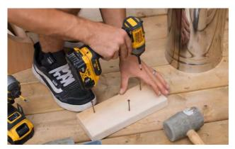
Place 3 – 3" (76mm) screws into each of the 3 chimney support boards.
