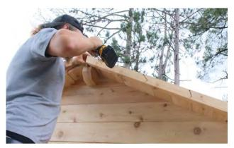
Pre-place 4 – 3" (64mm) screws into the front trim pieces and secure to the roof staves.
