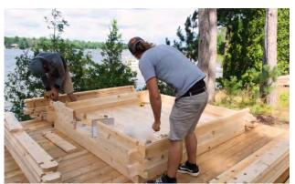
Continue with the front wall by placing one of the medium length wall staves on both ends and tapping them so the groove goes tight into the tongue of the front starter stave and secure it with a 5" (127mm) screw into the notch.
