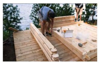
Fasten the front and rear starter staves with 2 - 3" (76mm) screws to secure it to the floor.
