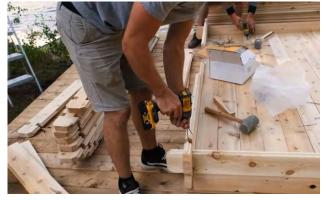
Insert a 5" (127mm) screw into the notch to secure it to the starter stave below.
