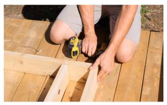
Insert 2 – 3" (76mm) screws into the end of each base stave.
