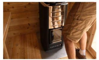
Place the stove onto the heat shield.
