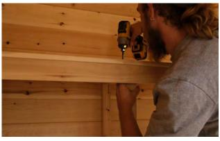
Align the bench supports to the slats on bottom of bench.
