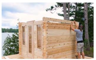
Insert a rear wall stave and a side stave on either side of the sauna and secure using 5" (127mm) screws into the notches on each end of the staves.
