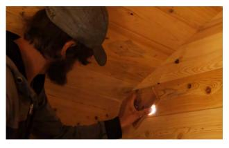
Use a 1  $\frac{1}{2}$ " (38mm) screw and attach the vent board on the inside of the sauna making sure it is tight but can still be turned.
