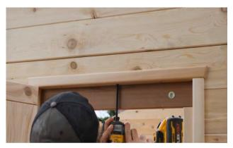
Use a 5" (127mm) screw in between the previously placed screws in the top of the door frame to pull in the middle of the triangle piece.
