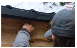
Secure the support to the wall lining up the center to the mark placed on the wall.
