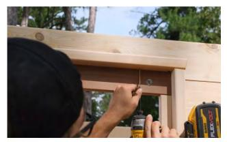
Insert 2 – 3" (64mm) screws into the top of the door frame as shown.
