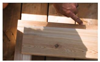
Ensure the "floor Starter" stave is flush with the inside of the front and side base plates.
