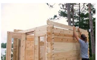
Place the side wall stave with the tapered edge on the side wall and secure in the notches with a 5" (127mm) screw on both sides of the sauna.
