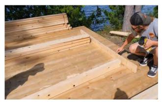
Start the assembly of your Georgian Cabin by laying out the front and back base plates and the 8 – base supports.
