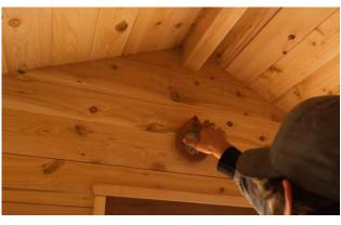
Install the optional Thermometer using a 1 ½" (38mm) screws.
