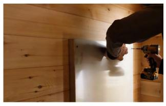
Secure the heat shield to the wall with 6 – 1" (25mm) screws.
