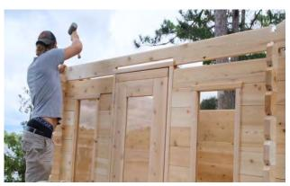
Secure the other full length front wall stave labelled "Door" above the windows and door and secure with 5" (127mm) screws into the notches in the same manner as the previous steps.
