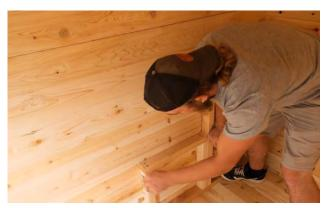
Start the assembly of your benches by placing the 2tier bench support along the wall.
