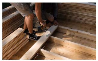
Secure with 2 - 3" (76mm) screws per support.
