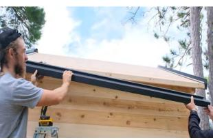
Place the long metal trim pieces on the sides of the roof and secure with the included short black screws.
