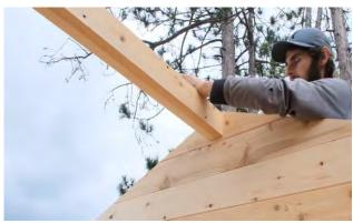
Place the center roof support beam into the slots on the top of the triangle pieces.
