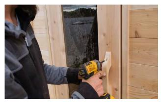
Install the outer door handle (small) at the desired height using 2 – 2 1/2" (64mm) screws in the pre-drilled holes.
