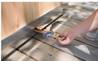
Using a pipe wrench or adjustable wrench, tighten the garden hose connector (if ordered) onto the valve.
