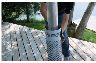
Remove the protective film from the chimney.
