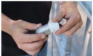
Screw the short pipe into the elbow.
