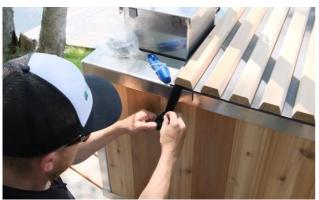
Place a locking clasp onto one of the straps at the end with the heater and pull it snug.
