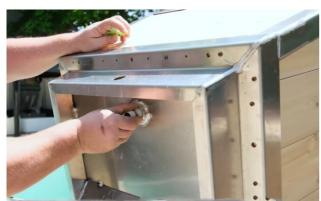
Thread the short nipple into the drain hole from the bottom of the cold plunge tub.
