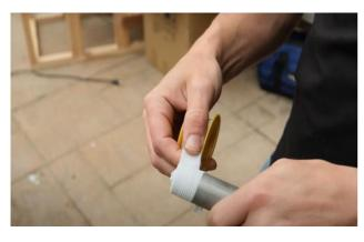
Wrap 3 layers of thread tape around the threads on both ends of the long nipple.
