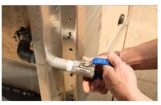
Screw the valve onto the end of the long nipple.
