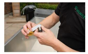
Wrap 3 layers of thread tape around the threads on both ends of the short nipple.
