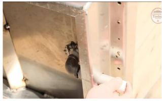
Thread the long piece of pipe into the elbow. This can be hand tight only at this time.
