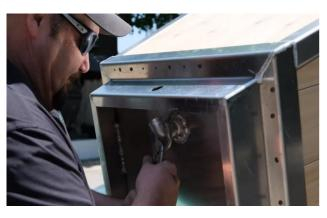
Screw the 90° elbow onto the short pipe.
