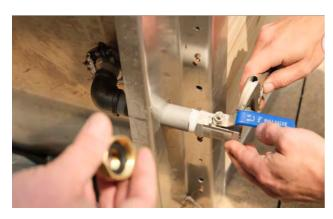
Using a pipe wrench or adjustable wrench, tighten the valve.
