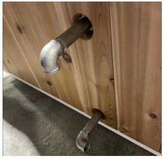
Thread an elbow onto each of the long pipes on the side of the tub.
