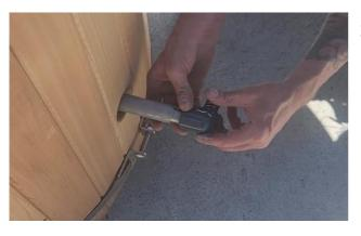
Screw one of the 90° elbows onto the bottom pipe of the cold plunge tub ensuring it is tight.
