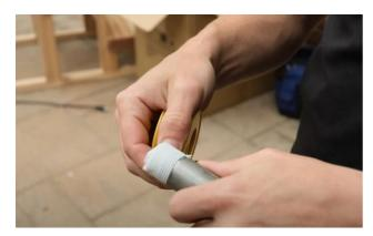
Wrap 3 layers of thread tape around the threads on both ends of the 2 long pipes.
