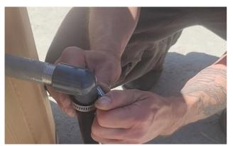
Connect a piece of tubing to the other side of the in-line strainer and secure with a hose clamp.
