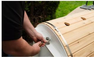
Screw elbow onto the short pipe ensuring it is tight and faces the back of the tub.
