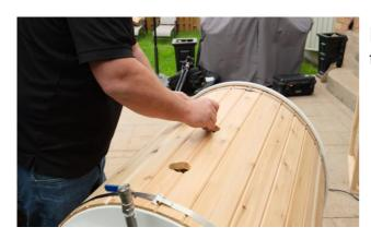
Remove the plugs from the holes in the side of the tub.
