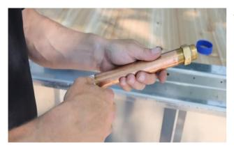
Wrap 3 layers of thread tape around the threads on both ends of the long pipe.
