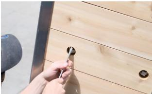
Remove the plugs from the holes in the side of the tub.
