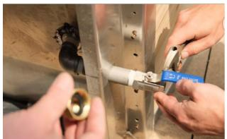
Using a pipe wrench or adjustable wrench, tighten the valve. This will also tighten the long adapter into the elbow. Have the handle of the valve facing in your desired position when tight.
