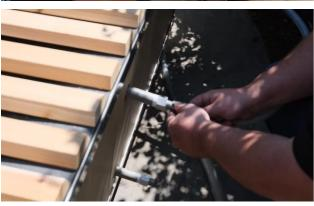
Connect the other ends of the chiller hoses to the tub. The hose from the outlet of the chiller will connect to the higher pipe of the tub and the hose from the inlet will connect to the lower pipe.
