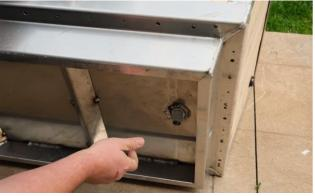
Thread the short piece of pipe into the drain hole from the bottom of the cold plunge tub. This can be hand tight only at this time.
