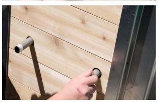
Wrap 3 layers of thread tape around both ends of the threads on the 2 remaining long pipes and thread them into the holes on the side of the tub. This only needs to be hand tight at this time.
