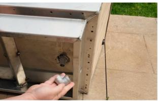
Screw the 90° elbow onto the short pipe. Ensure it is tight and facing the hole in the frame on the side of the tub.
