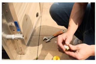
Wrap 3 layers of thread tape around the threads on the garden hose connector.
