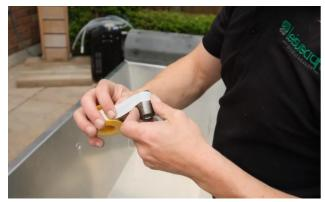
To start the installation of the cold plunge chiller, wrap 3 layers of thread tape around the threads on both ends of the short pipe.
