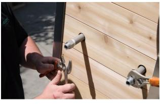
Screw the quick connects onto the pipes. Tighten with a pipe wrench or adjustable wrench.
