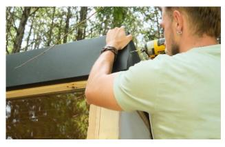
Place one black screw on the face of each side trim piece to tighten the seam with the front trim.
