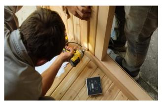
Place the 4-wire bundle into the groove of the wall trim and the 2-wire bundle out the bottom.
