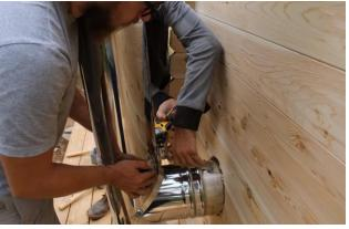
Attach the assemble chimney pieces to the "T" coming out the back of the sauna and secure with a support band.
