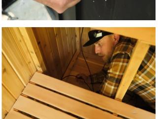
On the inside of the sauna, slide the wires along the wall under the lower bench and front enclosure to the front of the sauna where the heater and control panel will be located.
