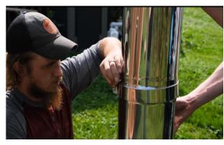
Attach the support strap around the 2 chimney pipes and tighten up.
