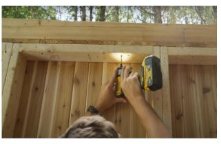
Repeat for the side wall panels ensuring the roof panel is flush to the side walls.
