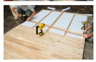
When you get to the middle of the floor, remove the temporary floorboard that was placed earlier.
