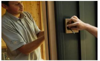
Feed the 4-wire bundle through the hole in the wall & control panel housing.
