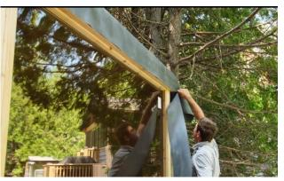
Cut off the excess membrane even with the nosing pieces and adding more staples as needed to get a tight fit.
