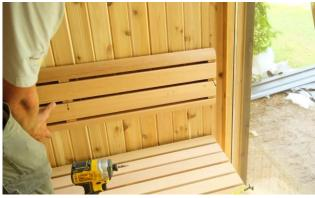
Place the side wall backrest 10" (25cm) to the bottom of the  $2^{nd}$  slat above the bench and secure with 2  $\frac{1}{2}$ " (64mm) screws into each support.
