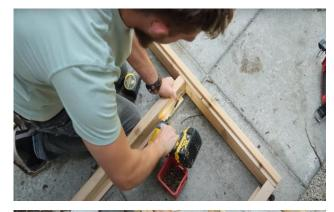
Space out the last floor joist and secure in the same manner as the previous joists.
