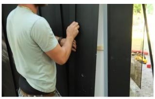
Remove the piece of metal siding to finish drilling the hole through the sauna wall.
