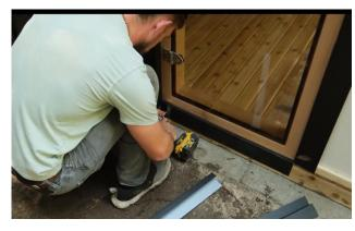
Place a short trim piece with the small lip below the door panel and secure with 3 of the provided screws.
