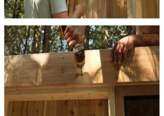
Secure the nosing to the roof panels with 9 – 2  $\frac{1}{2}$ " (64mm) screws.
