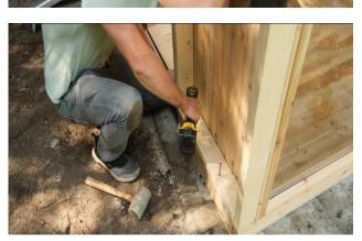
Once the front window is installed, secure the narrow panel on either side of the glass panel with 2 - 3 ½" (89mm) screws to the outside floor joists.
