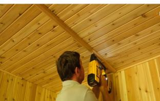
Measure the remaining gap and cut a piece to fit.
