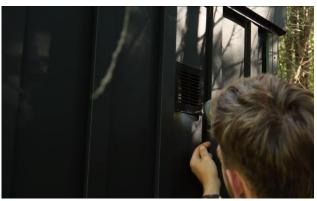
Install the vent and secure with the provided screws.
