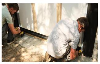
Install the bottom trim piece ensuring it is snug between the 2 side "J" trim pieces securing with 4 of the provided screws.
