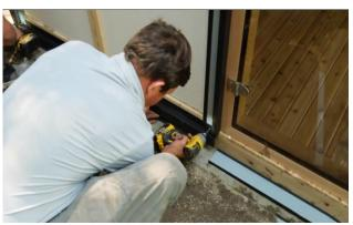
Install the bottom trim piece ensuring it is snug between the side "J" trim pieces securing with 3 of the provided screws.
