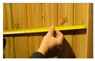
Measure 35" (89cm) from the front wall and 22" (56cm) up from the floor and mark it on the wall of the side you want the heater installed.
