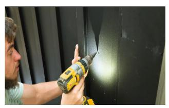
Drill a hole in the center of the 1st piece of metal siding on the back corner of the sauna to fit the plug for the wires.
