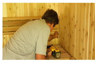
Measure the distance between the roof and the top of the backrest and from the backrest to the bench.
