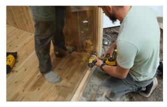
Use a 5/32" drill bit to predrill holes into the wall panels.
