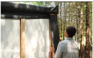
Repeat the process for the trim at the back of the sauna only securing with screws on the outside edges of trim at this point.
