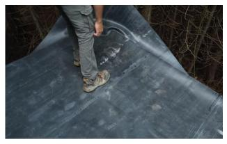
Spread the rubber membrane out evenly over the roof of the sauna allowing it to drape over the sides.
