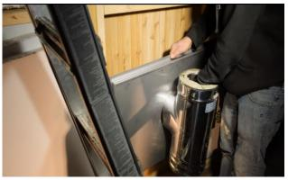
From the outside of the sauna, slide the chimney piece out and then put it through the exterior heat shield and then back into hole in the rear of the stove.
