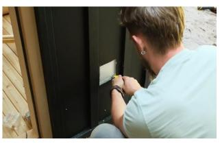
Repeat the process for removing the insulation and installing the vent for the lower vent hole.
