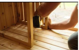
Ensure the bench is tight to the side wall then secure with 2 - 2  $\frac{1}{2}$ " (64mm) screws in the back support and 2 - 2  $\frac{1}{2}$ " (64mm) screws in the floor support on each bracket.
