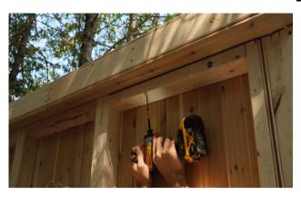
On the back wall of the sauna, locate the location of the studs in the roof panels by where the screws are.
