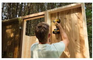
Install the last narrow next to the door and secure to the door panel with  $4 - 2 \frac{1}{2}$ " (64mm) screws.
