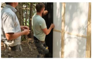
Place the first piece of metal siding by sliding it into the "J" side piece and then securing with 3 of the provided screws, 1 at the top, middle and bottom.
