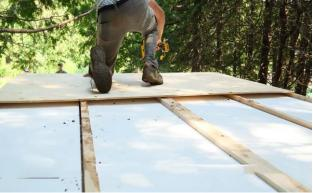
Ensure the plywood is flush to the front and sides of the sauna and secure with 1 ¼" (32mm) screws or staples.
