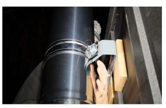
Attach the support strap to the chimney support and tighten bolts on both sides.
