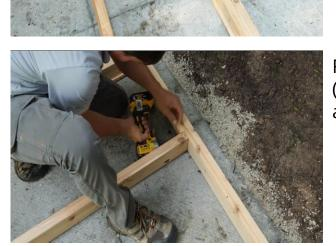
Fasten the floor joists to the back joist using 1 ½" (38mm) screws in the pre-drilled holes ensuring they are the same spacing as the front joist.
