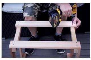
Screw heater guard support to either side using (2) – 1 ½" (38mm) screws per side.
