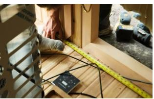
Measure the distance from the front of the lower bench to the trim piece and cut the other wire cover trim piece on a 45° angle at the measurement.
