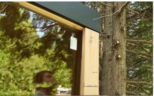
Place the first wood front trim piece on one side of the sauna front wall tight to the metal front trim.
