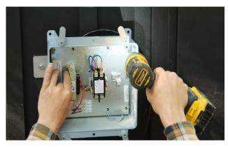
Secure the electrical components in the box and place on the cover.
