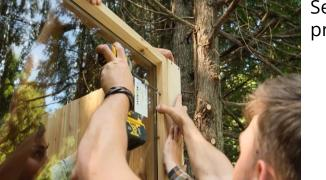
Secure the glass panel to the side wall panel with the provided lag screws ensuring the glass panel is flush.
