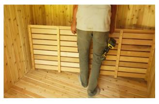
To start the assembly of the benches, bring in the large top bench and place it against the back wall ensuring the curved front of the bench is facing upwards.
