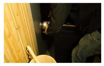
Place the stove on the floor shield then slide the chimney pipe into the hole on the back of the stove into the opening.
