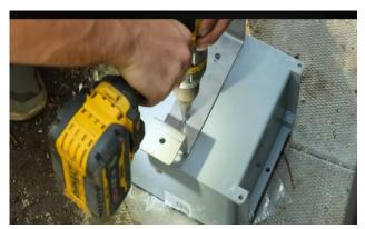
Flip over the box and bracket and drill out the mounting holes from the bracket into the electrical box.
