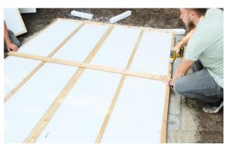
Secure a floorboard across the joists and secure with a 1 ½" (38mm) screw into each joist.
