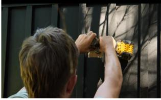
Drill a 2" (51mm) hole in the center of the cut out.
