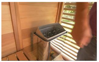
Hang the electric heater on the screws.
