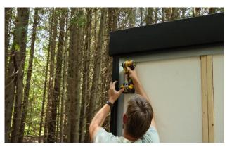
Place the side "J" piece next to the back trim and secure with 3 of the provided screws.
