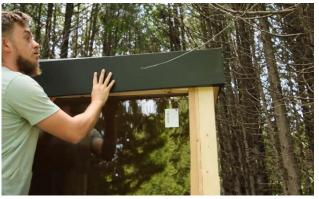
To start the installation of the metal trim, place the front metal trim piece over the front nosing.
