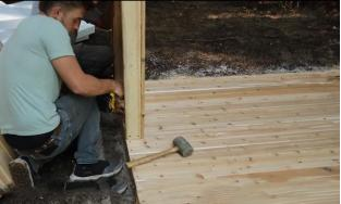
Ensure it is flush to the edge of the floor and secure with  $3 - 3 \frac{1}{2}$ " (89mm) screws into the outside floor joist.
