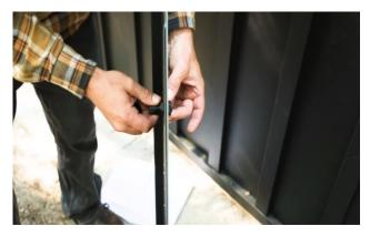
With the piece of metal siding removed, insert the plug through the hole and tighten with the plastic nut on the back of the siding.
