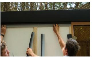
On the door side of the sauna, Place a top "J" piece between the trim piece and the door and secure with 3 of the provided black screws.
