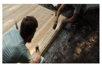
Do not fasten the last 3 floorboards to make it easier as you place the last smaller floorboard in to finish.
