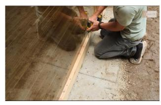
secure the front glass panel with 4 - 2  $\frac{1}{2}$  (64mm) screws to the front floor joist.
