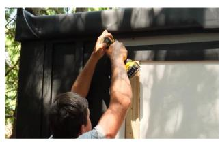
Install the next piece of metal siding, hooking it into the previous siding piece and secure with 3 of the provided screws.
