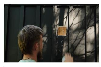
Using a utility knife, remove the insulation from the upper vent hole.
