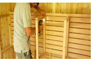
Repeat with the lower bench ensuring the curved front of the bench is facing upwards.
