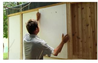
Start placing the insulation blocks into the wall panels.
