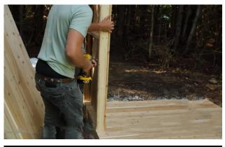
To start the assembly of the walls, bring a wide panel and place it on the back corner on the side of the sauna.
