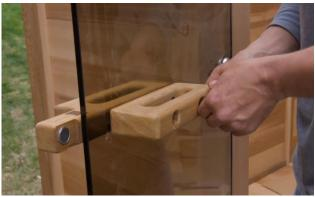
Ensure the outer handle lines up with the magnetic catch on the door frame and then tighten the lag bolts completely.
