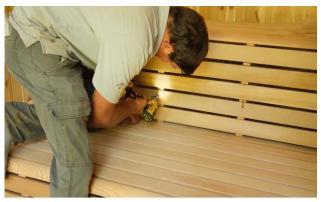
Place the upper bench enclosure in place and secure with 2 - 1 <sup>1</sup>/<sub>2</sub>" (38mm) screws into each support.
