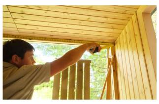
Measure the distance between the side walls at the seam above the glass wall and the roof.
