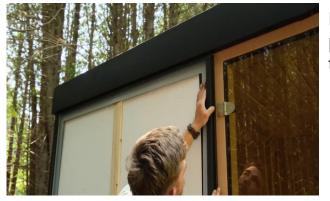
Place a trim piece with the small lip next to the door panel and a side "J" piece on top and secure with 4 of the provided screws.
