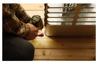
Secure the provided "feet" to the floor with the provided 1" (25mm) screws by sliding them under the heater and then pulling them back tight to the inside.
