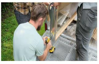
Install the panel rigger bracket onto the bottom sides of the window panel with the provided screws.
