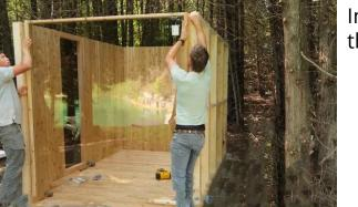
Insert the front window panel and ensure it is flush to the front of the floor and the side wall panels.
