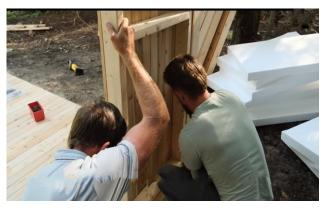
Place a narrow wall panel onto the back of the sauna and ensure it is flush to the base and the side wall panel.
