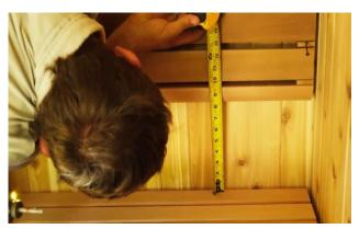
Place the large backrest 10" (25cm) to the bottom of the  $2^{nd}$  slat above the bench and secure with 2  $\frac{1}{2}$ " (64mm) screws into each support.
