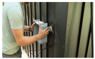
Position the electrical box on the bracket in your desired position.
