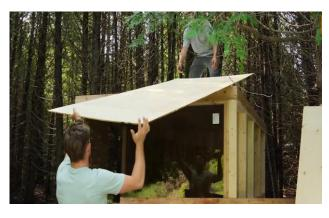
Place the first sheet of plywood onto the roof of the sauna.
