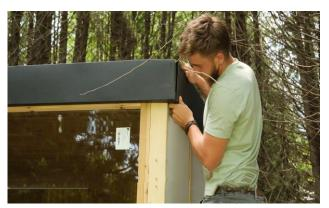
Place a side metal trim piece over the side nosing and secure with 6 black screws on the top and 3 centered on the bottom of the metal trim.
