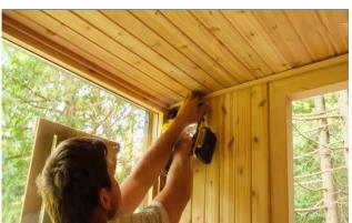
Use a full piece of the corner trim for the side wall. Measure the distance remaining and cut accordingly. Repeat on opposite side wall.
