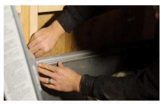
Level the exterior shield and mark on the outer studs where the mounting holes will be.
