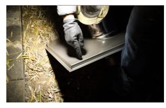
Measure the bottom mounting holes on the heat shield in relation to the top holes.
