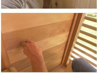
Install the supplied support screws into your marks as shown.
