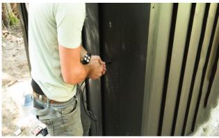
Feed the 2 wires through the plug, leaving a couple feed for the electrician to finish the hook up.
