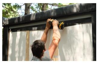
Starting at the back of the sauna, Place a top "J" piece between the 2 trim pieces and secure with 4 of the provided black screws.
