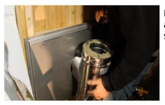
Place the heat shield and chimney back into position and secure in the corners with 4 of the provided screws.
