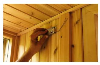
Remove the protective film from the temperature sensor cover and install over the sensor with 4 of the provided 1" (25mm) screws.
