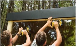
Fasten the trim to the nosing using 9 of the provided black screws.
