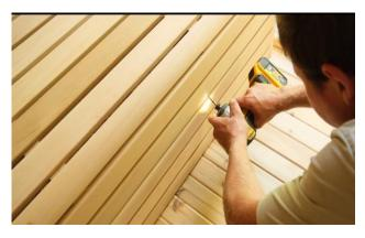
Place the side wall bench enclosure in place and secure with 2 - 1 <sup>1</sup>/<sub>2</sub>" (38mm) screws into each support.
