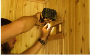
Place the cedar slider cover onto the bottom support then put the top vent support on top, ensure that the cover can slide back and forth.
