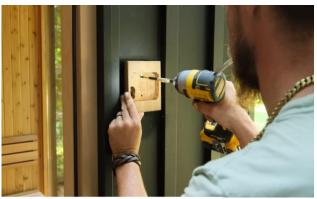
Secure the control panel housing over the hole with the provided screws ensuring it is level.
