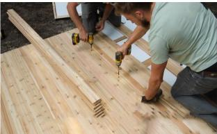
Secure the floorboards from this point to each floor joist with a 1  $\frac{1}{2}$ " (38mm) screw.
