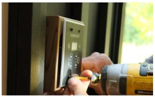
Secure the control panel to the housing block with the provided screws.
