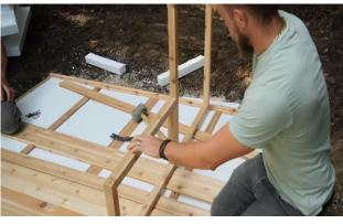
Once you get to 48" (122cm) from the rear of the sauna, place a screw in the floorboards where each of the joists are as they will be hidden by the benches.
