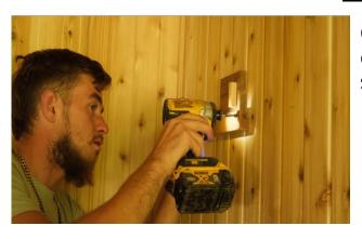
Center the bottom vent support under the hole, ensure it is level and secure it with 3 – 1 ½" (38mm) screws
