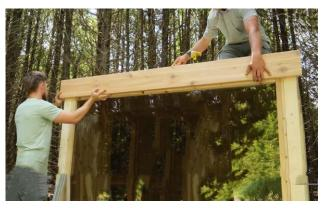
Repeat with the front nosing piece ensuring it is flush to the edge of the side nosing.
