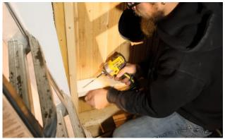
Transfer that measurement to the wall and secure another support in the same manner as the top support.
