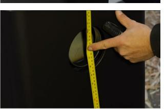
Measure the center of the chimney hole, in this case it is 22" (56cm)
