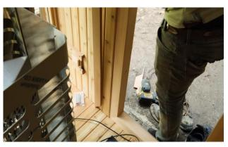
Measure the length of the wall beside the door and cut one of the wire cover trim pieces on a 45° angle at that measurement.
