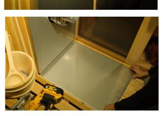
Place the floor heat shield centered to the wall shield.
