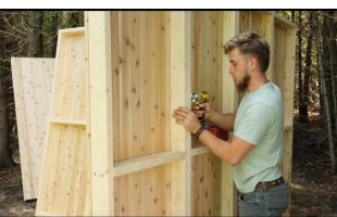
Repeat with 2 more narrow panels to finish the side wall ensuring the panels are flush to the edge of the floor securing with  $2 - 3 \frac{1}{2}$ " (89mm) screws into the outer floor joist and  $4 - 2 \frac{1}{2}$ " (64mm) screws into the previous wall panel.
