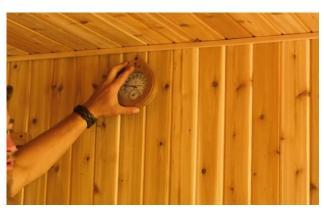
Use a 1 ½" (38mm) screw to hang the optional thermometer in the desired location.
