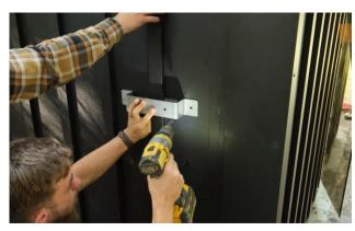
Place the support bracket for the electrical box and drill out the mounting holes.
