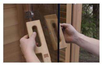
Install the door handle by placing the provided 2" (50mm) lag bolts through the inner handle (short)into the outer handle (longer)
