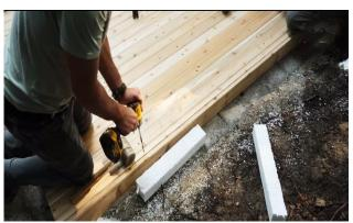
Once the last floorboard is in the proper placement, secure each of the unscrewed floorboards with a 1 ½" (38mm) screw into each joist.
