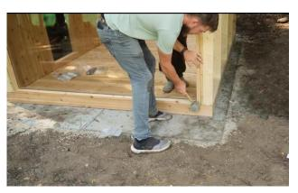
Use a rubber mallet to finesse widow until it is flush by tapping on the wood of the panel. (if needed)
