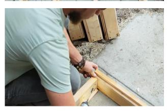
Secure the outside joists to the front and back joists using  $2 - 1 \frac{1}{2}$ " (38mm) screws per corner.
