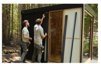
Follow the same process as the back wall for installing the metal siding pieces up to the door.
