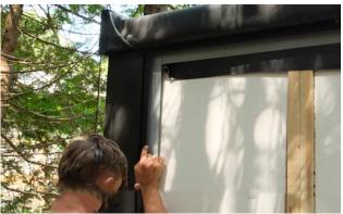
Place the side "J" piece next to the side trim and secure with 3 of the provided screws.
