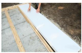
Place the blocks of foam insulation in between the joists.
