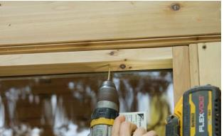
Use a 5/32" drill bit to predrill 2 holes from the glass panel into the roof panel.
