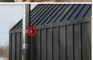
Attach the assemble chimney pieces to the "T" coming out the back of the sauna and secure with a support band.
