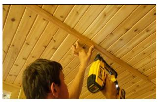
Install the crown molding over the seam between the 2 roof panels.
