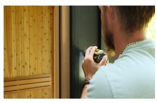
To start the installation of the floor model heater, drill a ½" (13mm) hole beside the door at the desired height where the control panel will be mounted.
