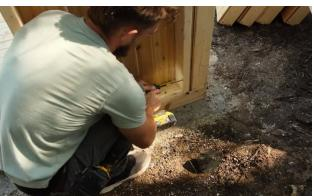
Ensure it is flush to the back edge of the floor and secure with  $2 - 3 \frac{1}{2}$ " (89mm) screws into the back floor joist and  $4 - 2 \frac{1}{2}$ " (64mm) screws into the other wall panel.
