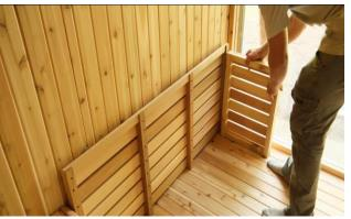
Secure the slotted bench support to the bench seat with 2 - 2  $\frac{1}{2}$ " (64mm) screws.
