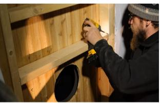
Remove the shield and chimney and secure the support with  $2 - 3 \frac{1}{2}$ " (89mm) screws in each end.
