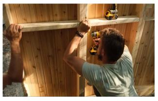
Repeat the process for 2 more narrow panels on the back wall ensuring they are flush to the back of the floor and to the previous panel.
