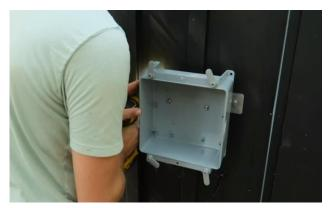
Mount the assembly to the wall with the provided lag screws.
