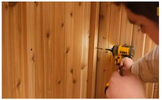
Ensure the bench is tight to the back wall then secure with  $2 - 2 \frac{1}{2}$ " (64mm) screws in the back support and  $2 - 2 \frac{1}{2}$ " (64mm) screws in the floor support on each bracket.
