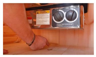
Locate a suitable location to drill a hole for the power cable.
