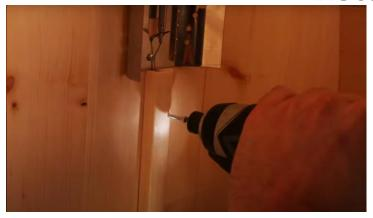
Use the pre-drilled holes in the trim pieces to avoid hitting the wires.
