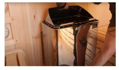
Remount the heater onto the screws
