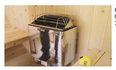
Hang the heater on the screws ensuring the heater is level and the bottom of the heater is 5-7" (13-18cm) above the floor.
