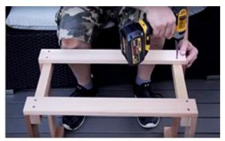
Screw the heater guard supports to either side using  $(2) - 1 \frac{1}{2}$ " (38mm) screws per side.
