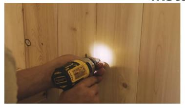
Install the two  $\frac{1}{2}$ " (6mm x 38mm) hex head lag screws (supplied with the heater) into the marks leaving them protruding from the wall  $\frac{1}{2}$ " (6mm).
