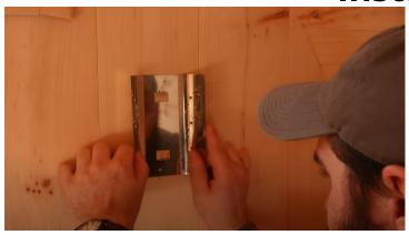
Secure the sensor housing to the wall with the provided screws.
