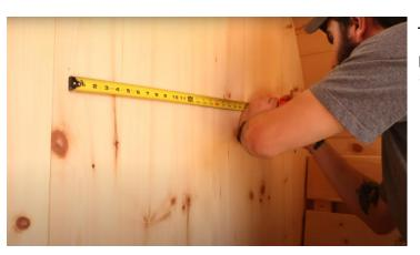
To mount the temperature sensor, measure and mark the wall 14" (36cm) from the heater and 14" (36cm) from the ceiling.
