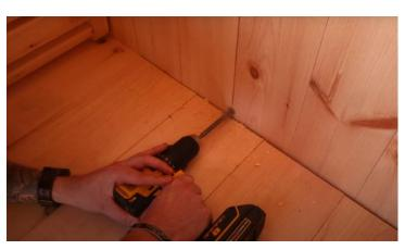
Use the 1 1/8" (29mm) drill bit to drill a hole through the wall.
