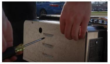
Lay the heater on its back and remove the screws securing the panel.
