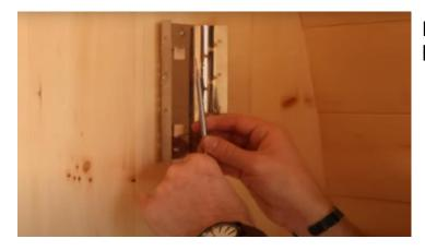
Insert the sensor into the grooves on the housing ensuring it is snug.
